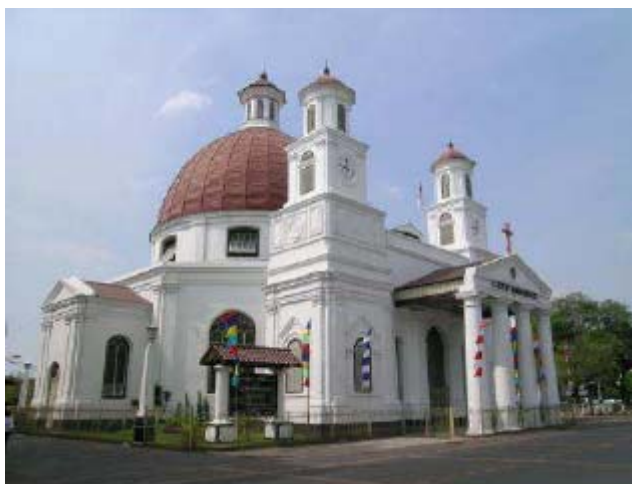
Figure 1 : Blenduk church view with twin towers
